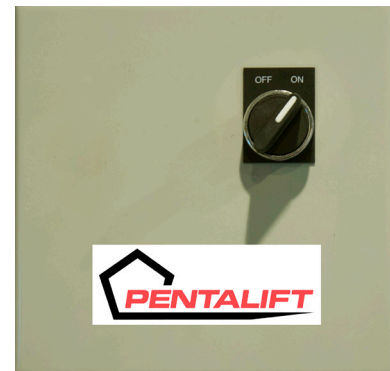
Control Panel 115/1/60 supply is transformed to 12 volt for lights
